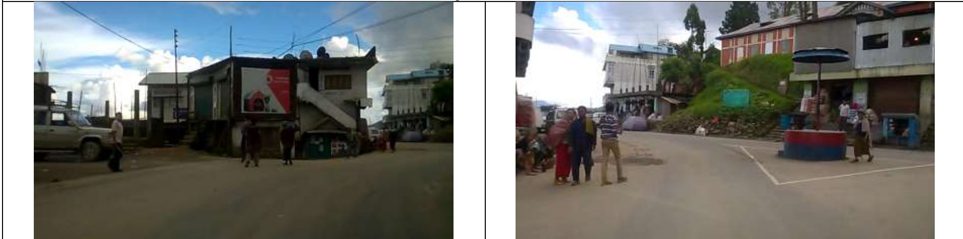
Photos at Mao (Km 213+000)
