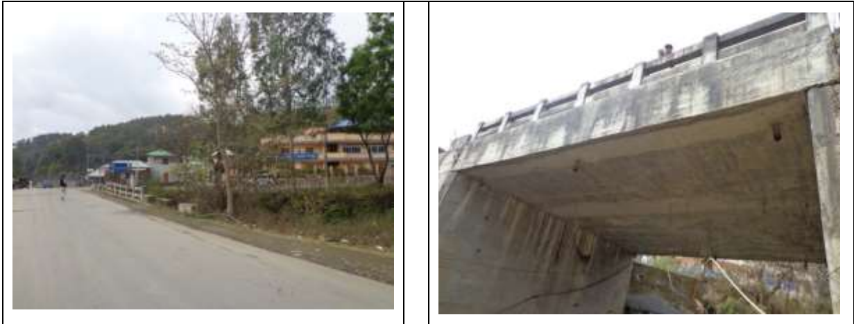
Minor Bridge at Km288+621
