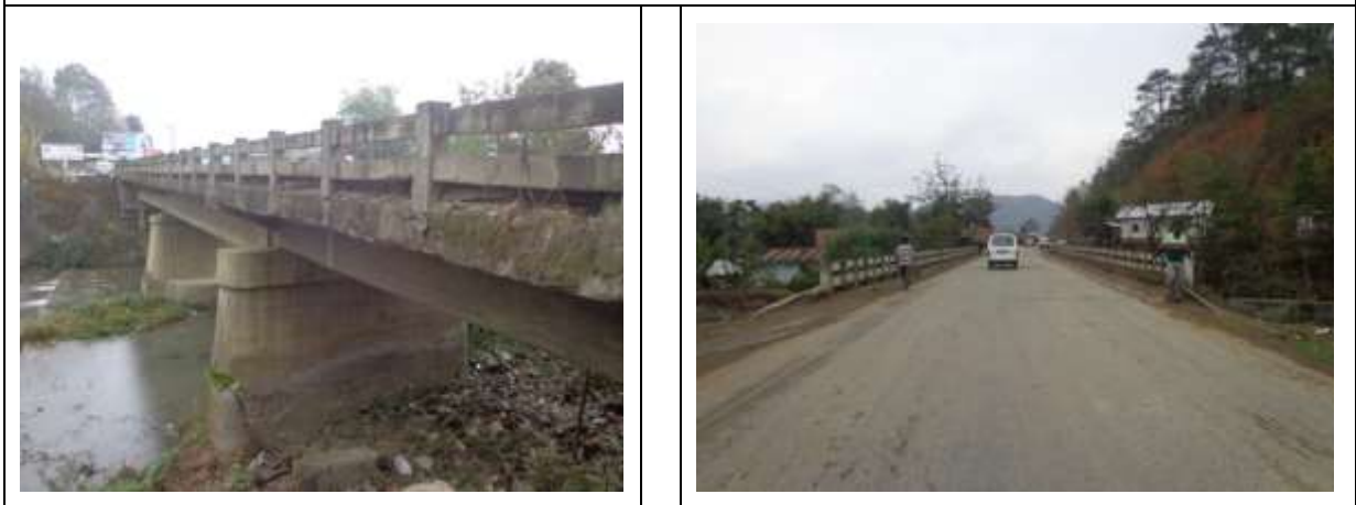
Minor Bridge at Km305+629
