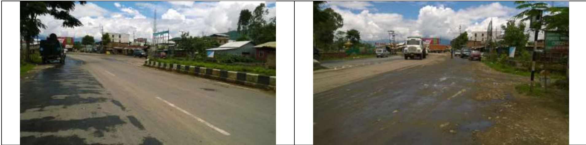
Photos at Project End (Km 311+082)
